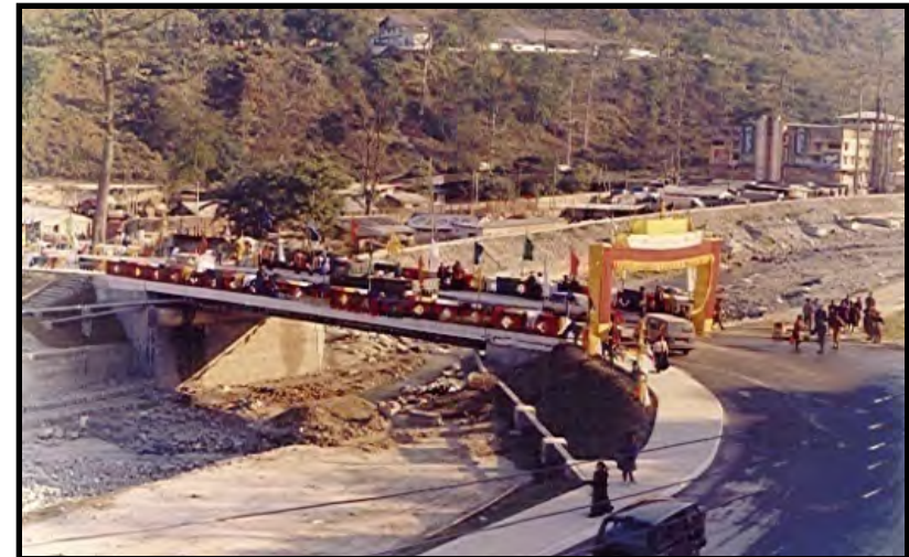
Construction of Dhutikhola Bridge at Phuentsholing, Bhutan
