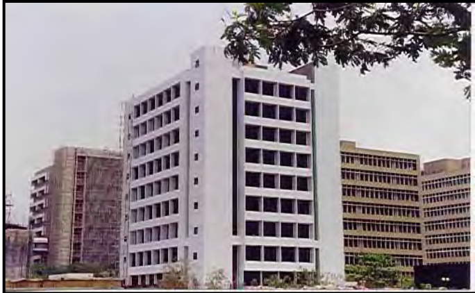
Construction of Office Building at Bandra-Kurla Complex for MMTC, Mumbai
