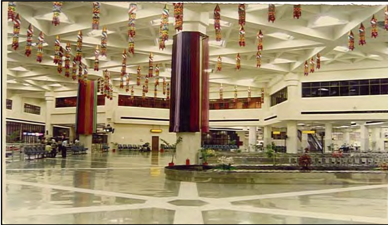
Construction of Airport Terminal Complex Building including Structural, Electrification and Finishing Item at Kolkata
