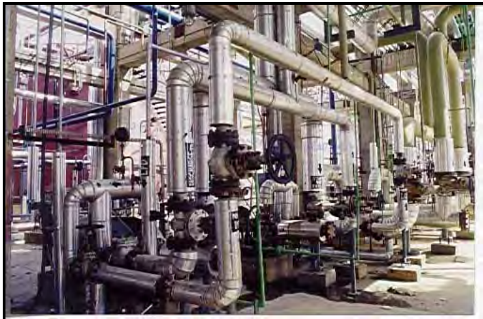
Unit Piping Work at Panipat Refinery Project for IOCL
