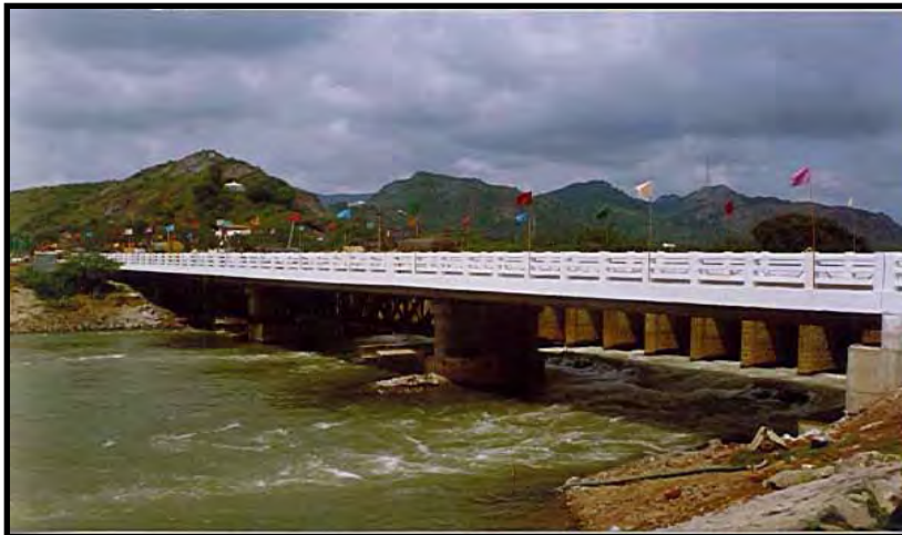
2 Nos. PSC Bridges on 2 Lane Highway of NH-9 at Vijayawada, A.P.
