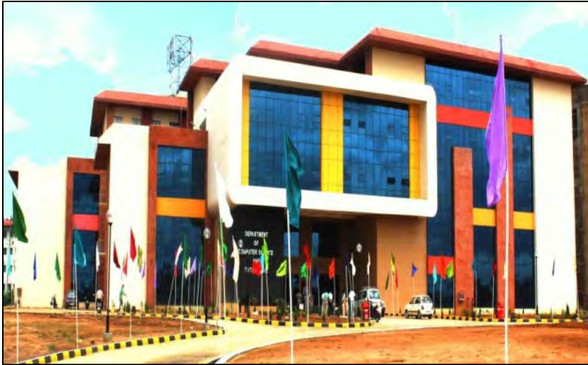
Construction of Computer Centre and Central Library at NIT, Agartala , Tripura
