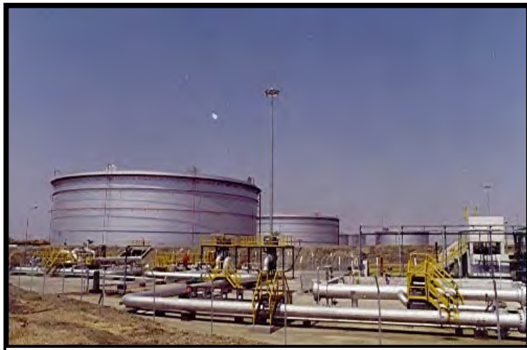
Turnkey Execution of 42,850 KL Oil Terminal for HSD, MS & SKO for IBP at Panipat
