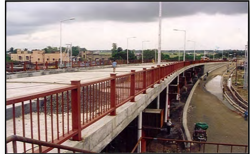
Construction of Flyover across NH-2 at DSP Main Gate Junction
