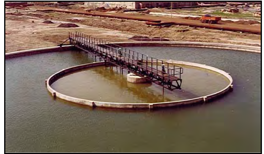
Clariflocculator with Bridge at Raw Water Treatment Plant for IPCL at Dahej
