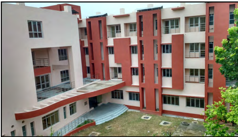
Construction of Hostel Building and Transit Quarter Complex for Satyendra Nath Bose National Centre for Basic Sciences , Kolkata
