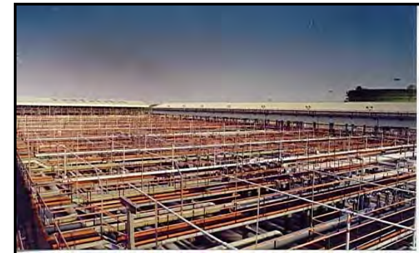
Yard Piping at Panipat Refinery Project for IOCL
