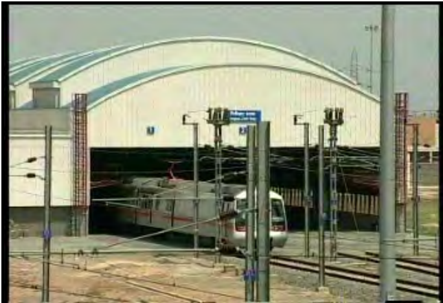
Construction and Commissioning of Khyber Pass Depot and workshop including property development deck work for Delhi Metro Railway Corporation
