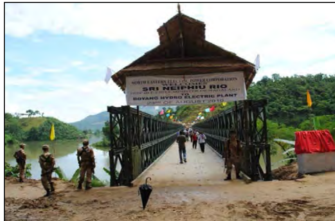
Asia's 2nd Longest Bailey Type Unit Bridge (3 X 200FT.) AT NEEPCO LTD., Nagaland
