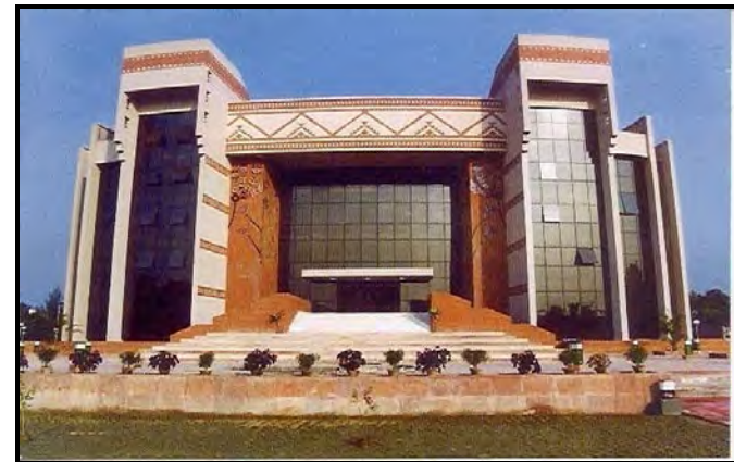
Construction of Auditorium and allied work at Indian Institute of Management, Joka, Kolkata
