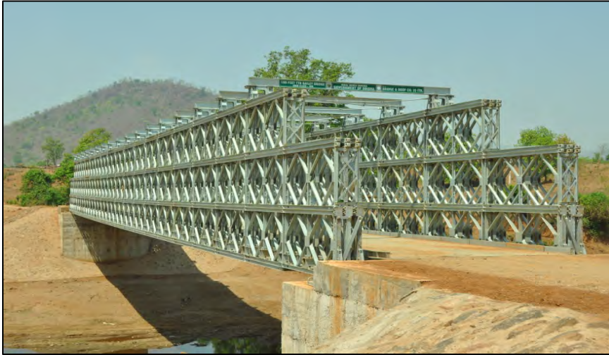
Construction Of Bailey Type Unit Bridge for Government of Odisha at various locations
