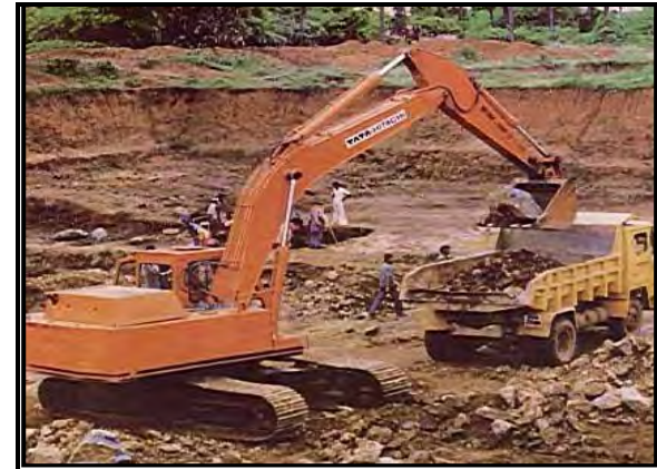
Area Grading Work at MRPL Mangalore
