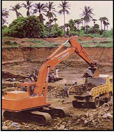
Excavator-cum-Loader and Dumper
