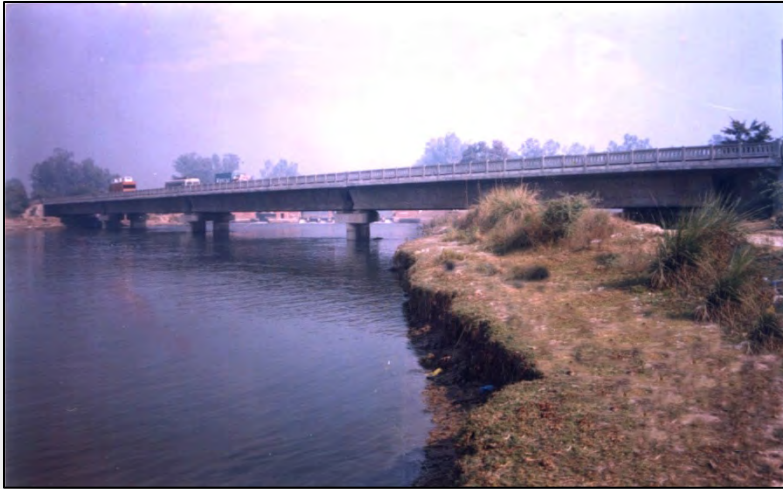
PSC Bridge 4 Lane Bridge at Karnal on NH-1 including Design For PWD/Haryana
