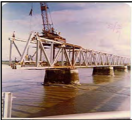
Bridge over Mahananda River for Indian Railway
