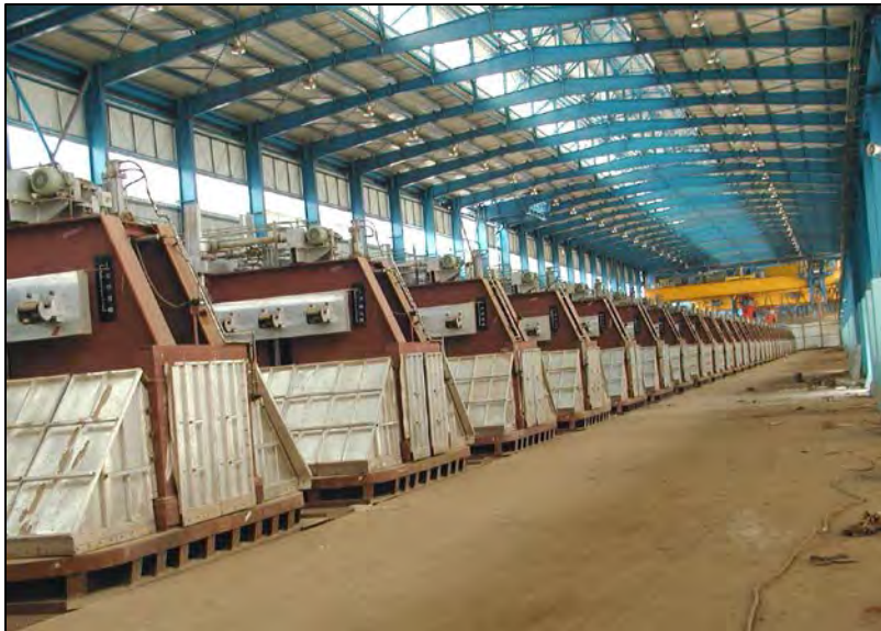
Civil & Structural Works in Potline Area at BALCO Korba
