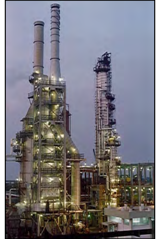
VDU Furnace at IOCL, Haldia
