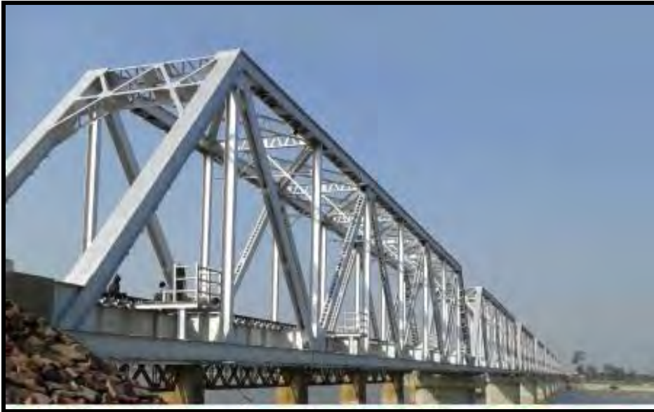
10 X 61m span Rivetted Type Through Bridge Girders on Bareilly Kasganj section for North Eastern Railway
