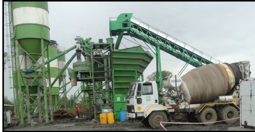
Batching Plant and Transit Mixer
