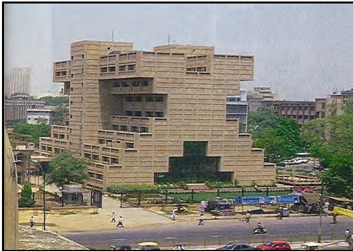
Civil, Sanitary & Land Scaping work of Golden Jubilee Building of Indian National Science Academy, New Delhi
