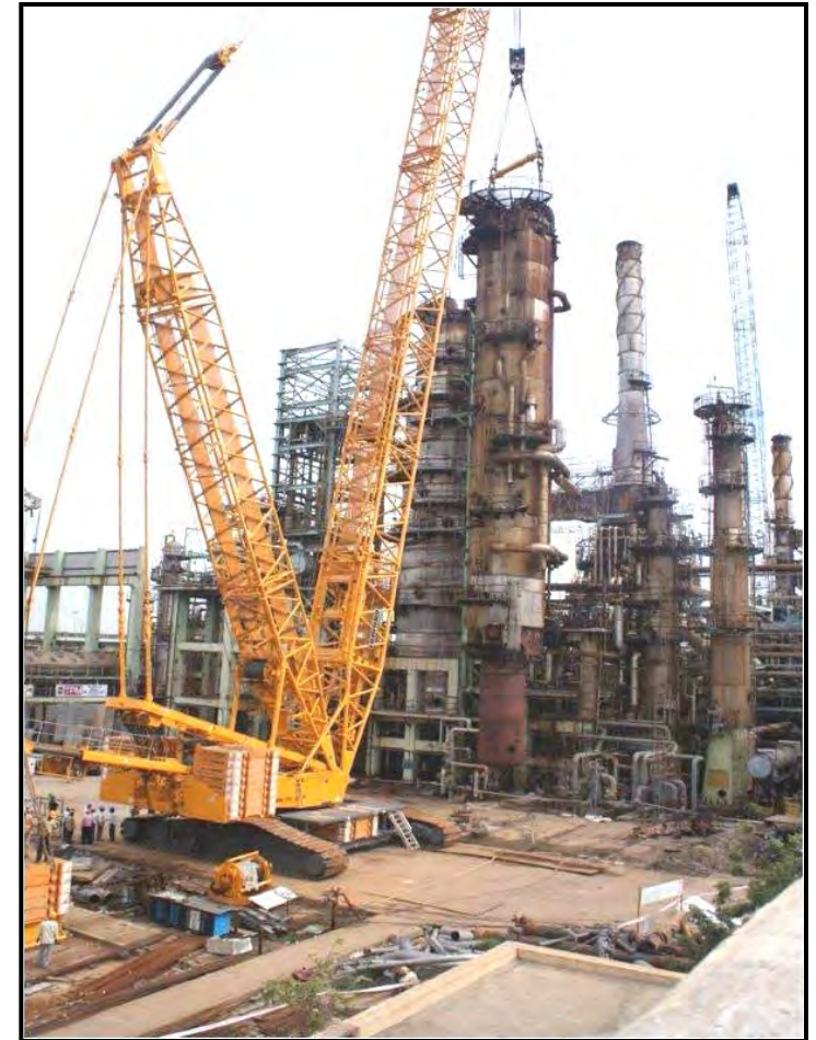
CDU / VDU - II Revamp Project in Chennai Petroleum Corpn. Ltd.
