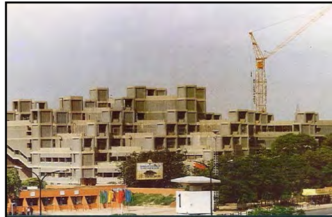
National Science Centre at Pragati Maidan, New Delhi complete sub-structure i/c Piling, Basement, Super Structure work, Sanitary, Plumbing & Fire Fighting work
