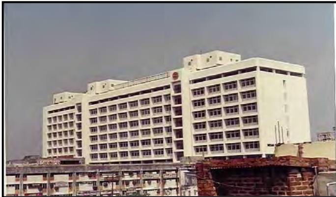
General Building work & Sanitary & Plumbing work including Fire Fighting Arrangement for IOCL Office Block at Kolkata
