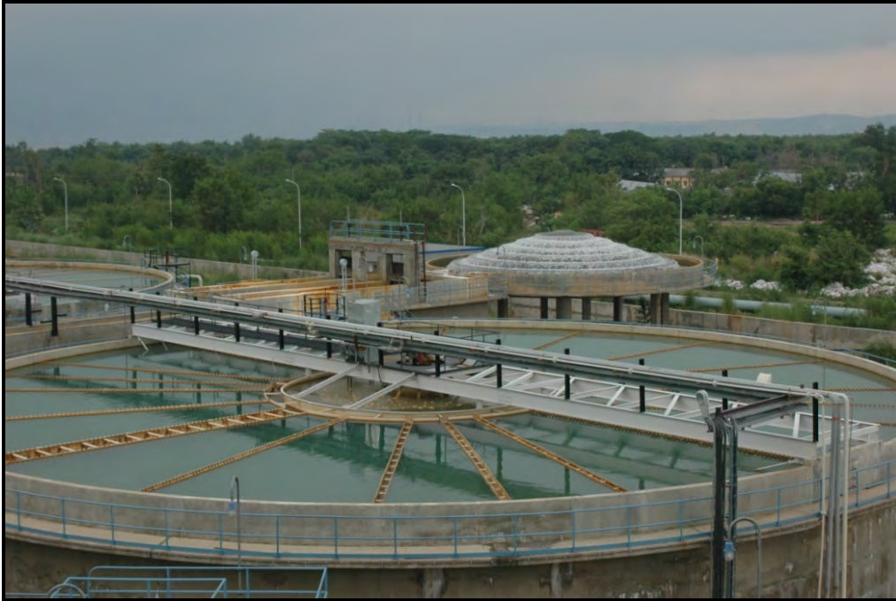
Pre-Treatment Plant, Raw and CW Make-up Water System Package for Rihand Super Thermal Power Project Stage-II of National Thermal Power Corporation Ltd.
