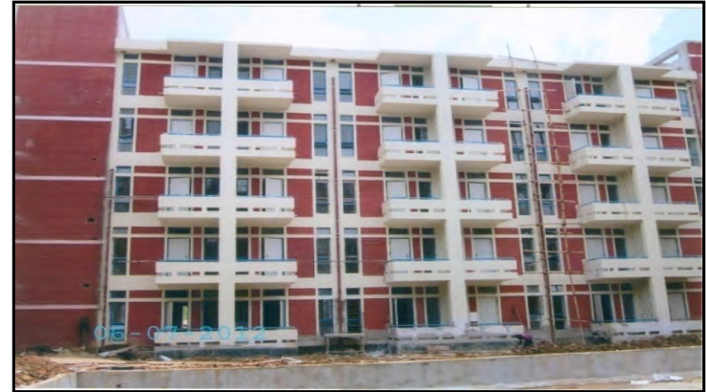
Construction of 2000 capacity Boys Hostels including 1000 capacity Dining Hall at IIT Kharagpur , West Bengal.
