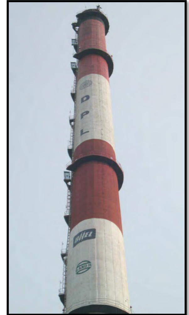
Construction of 220 M high RCC single flue brick lined chimney for 1 X 250 MW Unit at Durgapur Projects Ltd. for BHEL
