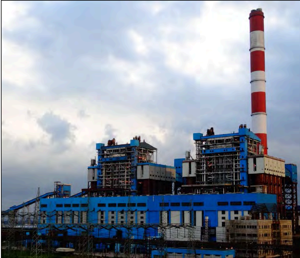
Civil & Structural work for Power Block Unit at 2X500 MW Unit # 1 & 2 at Durgapur Steel Thermal Power Station of Damodar Valley Corpn. at Andal
