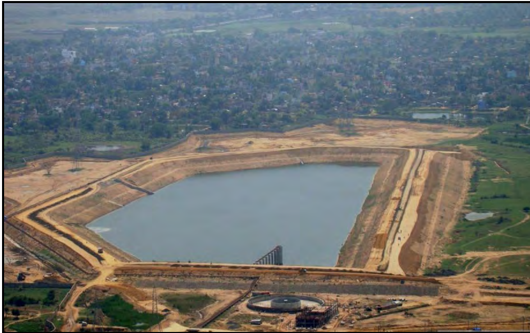
Ash Disposal at 2X500 MW Unit # 1 & 2 at Durgapur Steel Thermal Power Station of Damodar Valley Corpn.
