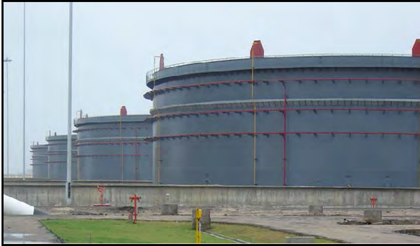
Double Deck Floating Roof Tank, 79 Mtr. Dia. X 13.5 Mtr. Ht. at Mundra of M/s. IOCL
