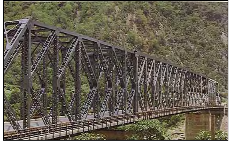
2x50m & 1x100m, 2 lane Road Bridge over River Tamur in Nepal
